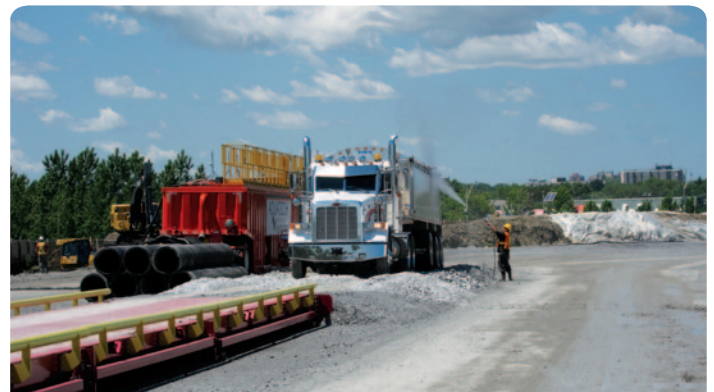
Soil Removal Operation
